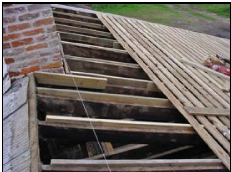
The photo at right shows the roof above the plantation office of Lakeport Plantation house. The roof was deteriorated and the original skip sheathing had to be replaced with new. The damaged rafters shown here were straightened and braced with new materials as well.
