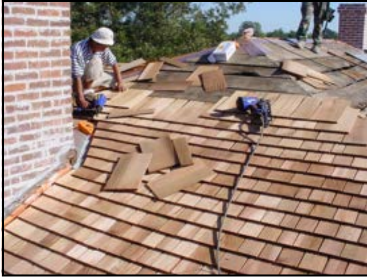
The photo at left shows the new cedar shingles being put on the roof of Lakeport Plantation house. Cedar shingles were used instead of cypress because of the high cost of cypress shingles.
