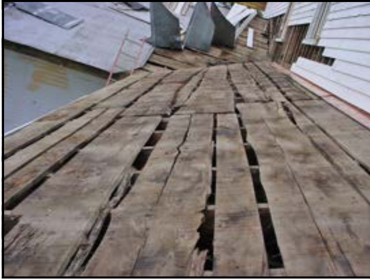
The photo at left shows the original cypress skip sheathing that was exposed when the corrugated metal roof was removed. Crudely cut, many of the boards still have the barked edges and are shaped like the trunk of the trees from which they were cut.
