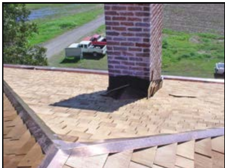
The photo at right shows the copper flashing covering the ridges of the roof of Lakeport Plantation house. The flashing is used to protect the roof in areas where the shingles cannot; along the ridges, at the hip and in the valleys of the roof.
