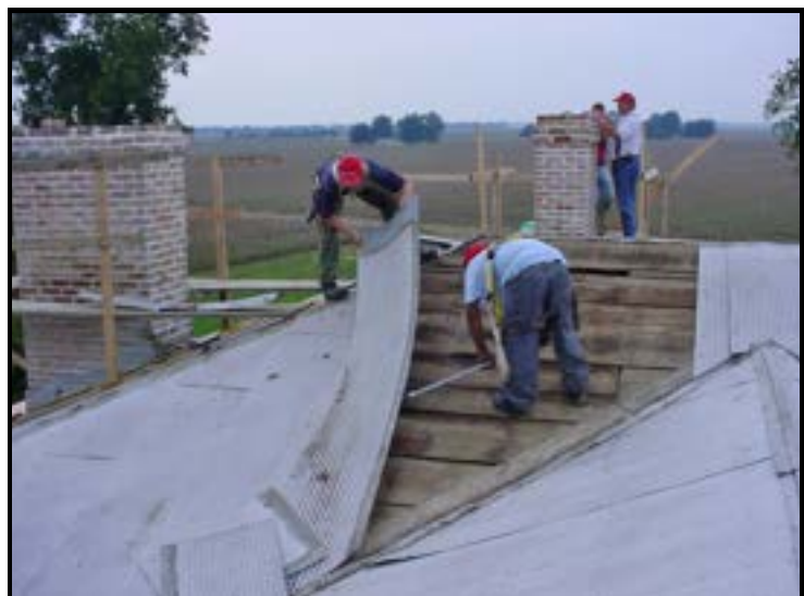
The photo at right shows the restoration crew removing the corrugated metal roofing material from Lakeport Plantation house to get ready for the new cedar shingles to go on.
