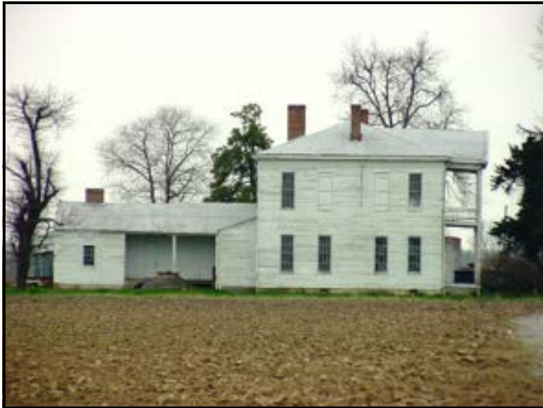
This photo shows the south side of Lakeport Plantation house before restoration began. At that time, the hip roof was covered with a corrugated tin roofing material.
