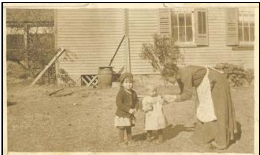
The historic photo at right shows the original latticework that was built between foundation piers at the back of Lakeport Plantation house. This photo was provided by descendants of the Johnson family.
