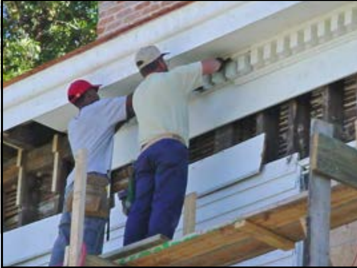
The photo at left shows Lakeport restoration workers putting up new dental molding on the west side of the house. The dental molding on this side of the house had been removed in earlier years and was never replaced.
