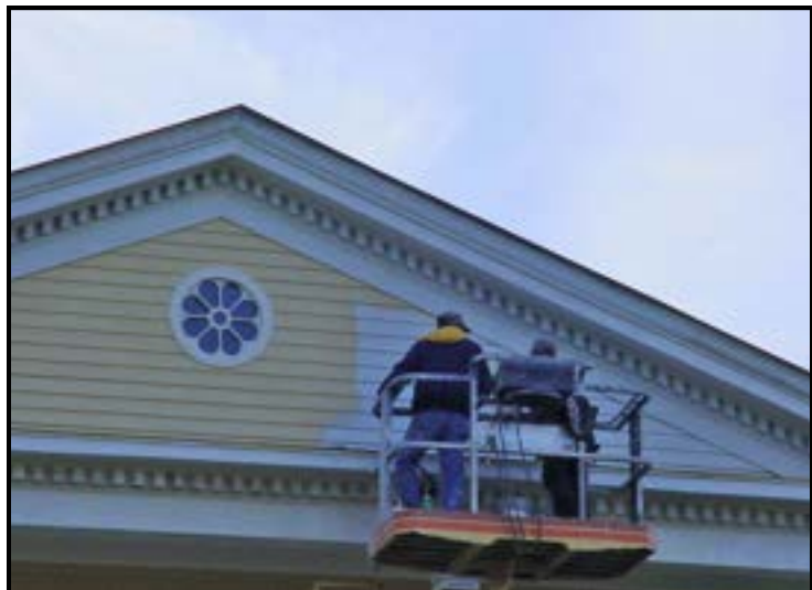
The photo at right shows the front porch pediment receiving a coat of paint. The paint color, a reproduction of the original, emphasizes the intricate detailing of the newly restored rose window.
