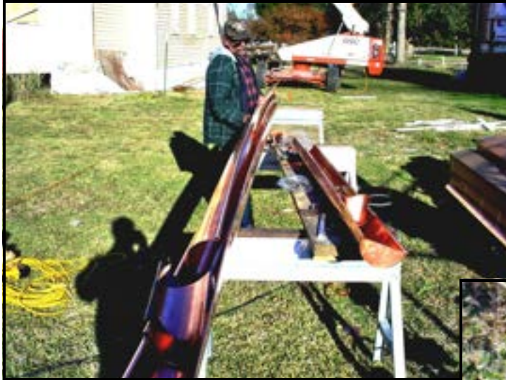
These photos show the fabrication of the half-round copper gutters that were installed on the ell part of Lakeport Plantation house.
