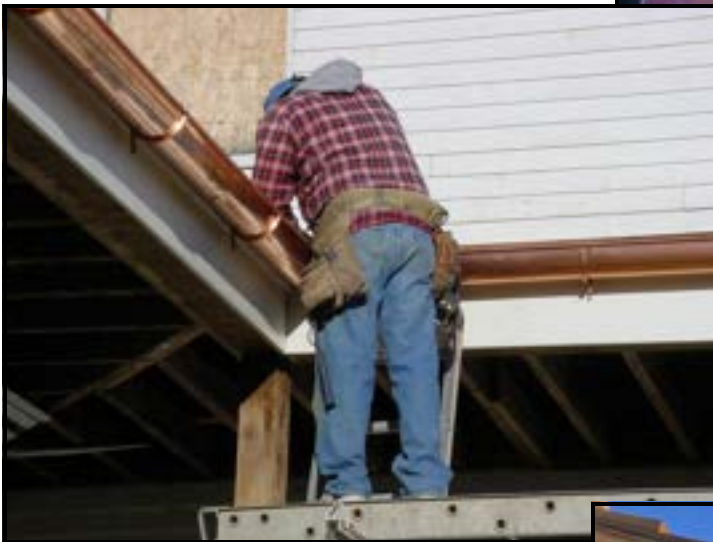
The photo above shows the half-round gutters being installed on the inside corner of the ell porch. The photo at right shows the beginning of a downspout that has been fabricated and attached to a half-round copper gutter.
