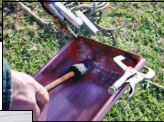
The photo at left shows sections of the half-round gutters being readied for installation. The photo below shows an end piece being soldered to a half-round gutter.
