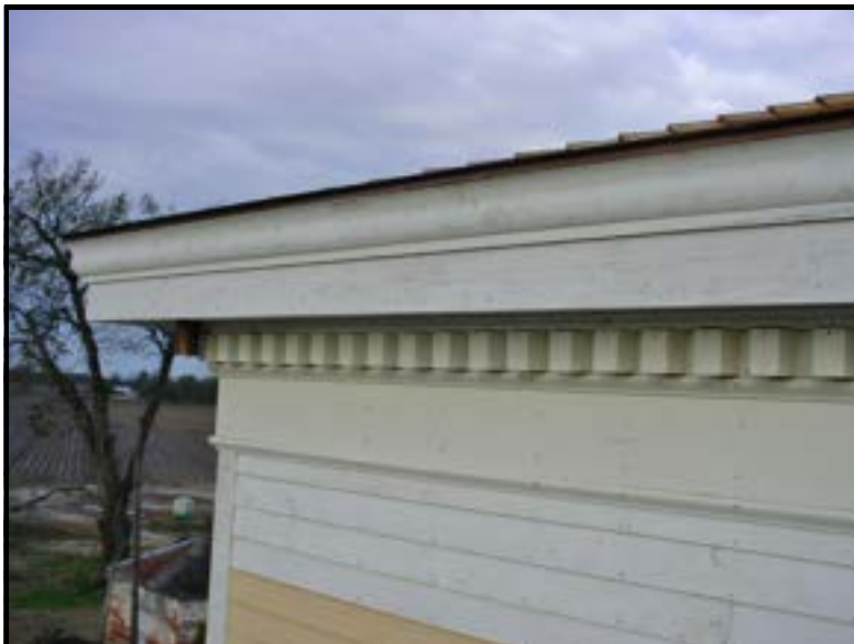
The photo at left shows the cornice molding that hides the box gutters on Lakeport Plantation house. Built-in gutters provide water drainage without interfering with the architectural details of the house.
