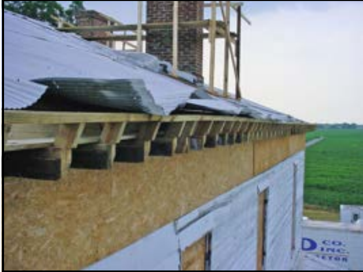
Most of the original box guttering was gone when restoration began and what remained was removed and replaced using new materials. This photo shows the new frame that was built along the west wall of Lakeport Plantation house to hold the new box gutters.
