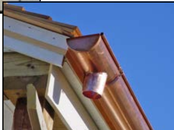
The photo above shows the half-round gutters being installed on the inside corner of the ell porch. The photo at right shows the beginning of a downspout that has been fabricated and attached to a half-round copper gutter.
