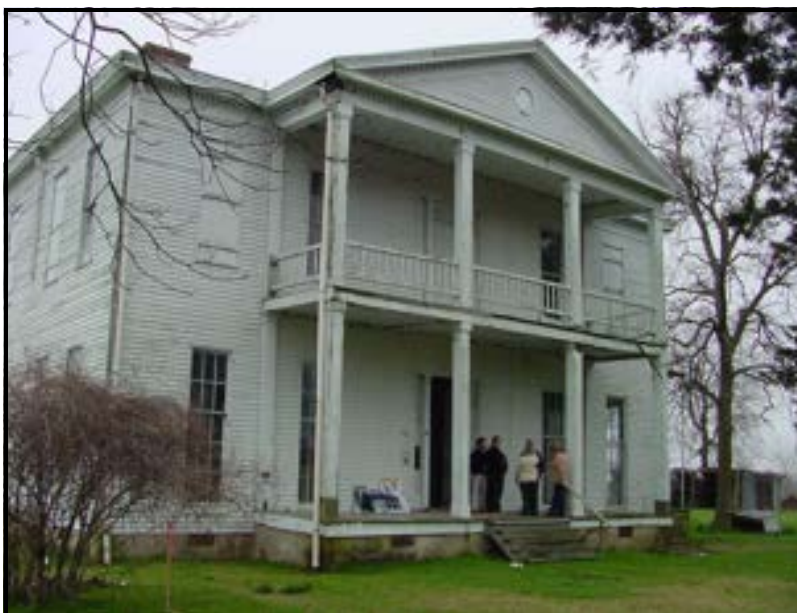
The photo at left was taken in March, 2003, as restoration was beginning. At that time, Lakeport Plantation house was approximately 140 years old. The braced frame method of construction used to build Lakeport had kept the house straight and strong through the years.
