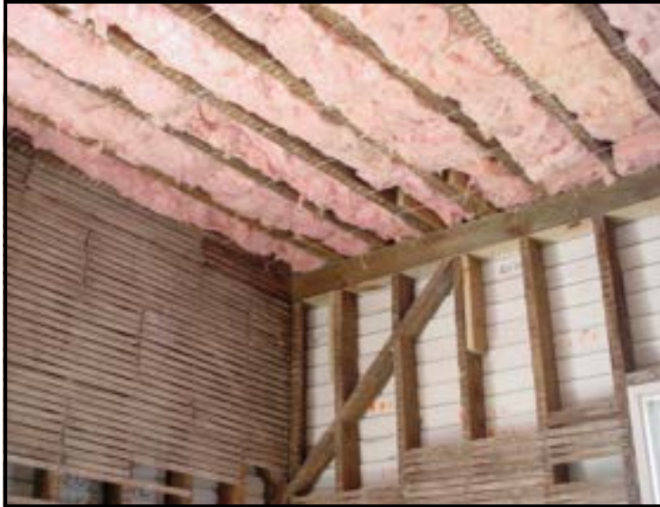
The photo at left shows the braced frame construction from the interior of Lakeport Plantation house. Seen in this photo is a corner brace, wall studs and top plate beam as well as ceiling joists for the plantation office. The siding that covers the framing on the exterior and the plaster lathing that covers the framing on the interior can also be seen.
