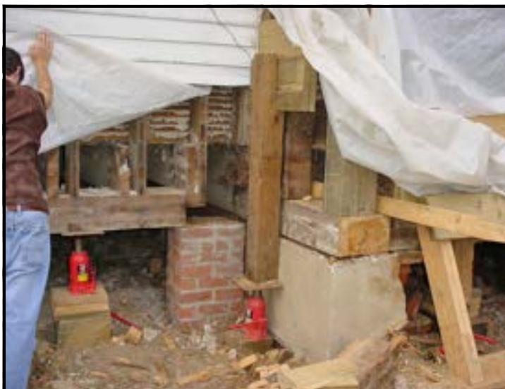
The photo at left shows the framework of Lakeport Plantation house being lifted with the used of hydraulic jacks as the foundation walls were being rebuilt. The foundation walls had collapsed in several areas causing the framework of the house to sag.
