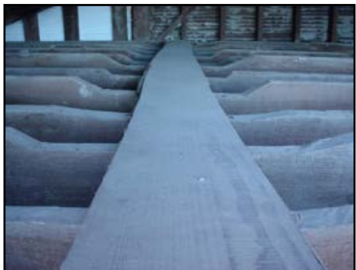
This photo was taken in the attic above the plantation office. The center board, called a rat run, is used to tie the ceiling joists together. The boards used for the ceiling joists were all different widths and had to be cut away in the center at different depths for the rat run to lay level.
