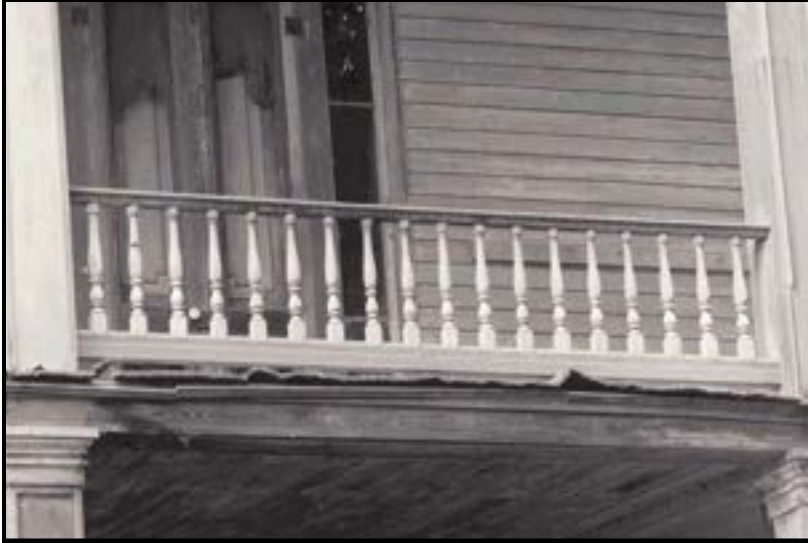
The photo at left shows the original front porch balustrade as it was around 1925. This historic photo was taken from the Lakeport Plantation Historic Structures Report.
