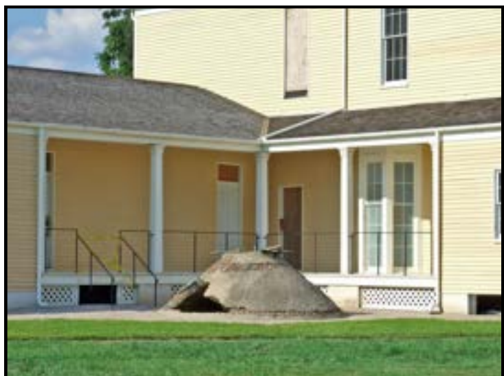
The purpose of the ell porch was strictly functional, providing sheltered access from the main house to the kitchen and commissary. Of simple design, the one decorative element is the bay window that holds opaque patterned glass window panes.
