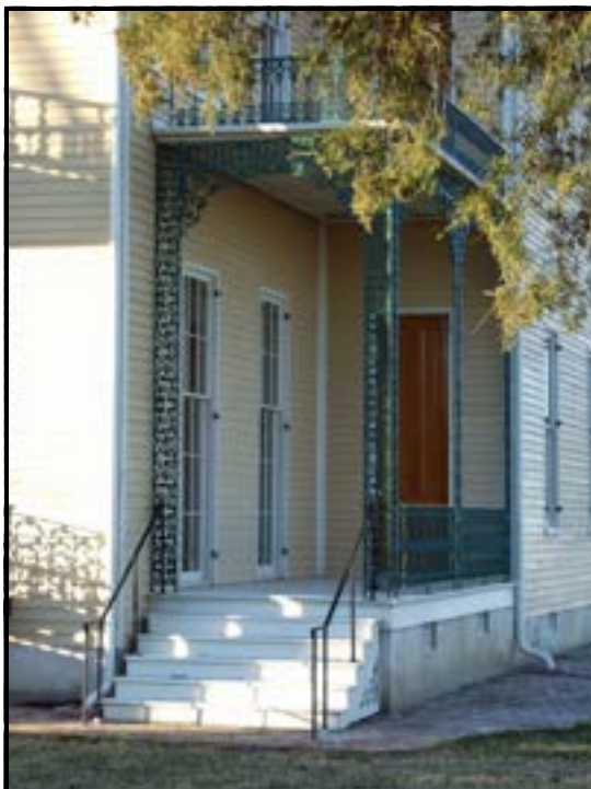
The photo at left shows wooden steps that were built for the ornamental iron porch. Wood steps with closed treads were built for all of the porches of Lakeport Plantation house.
