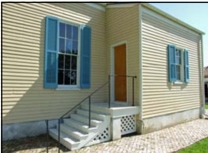
The small stoop provides another access to the plantation office from the north side of Lakeport Plantation house.
