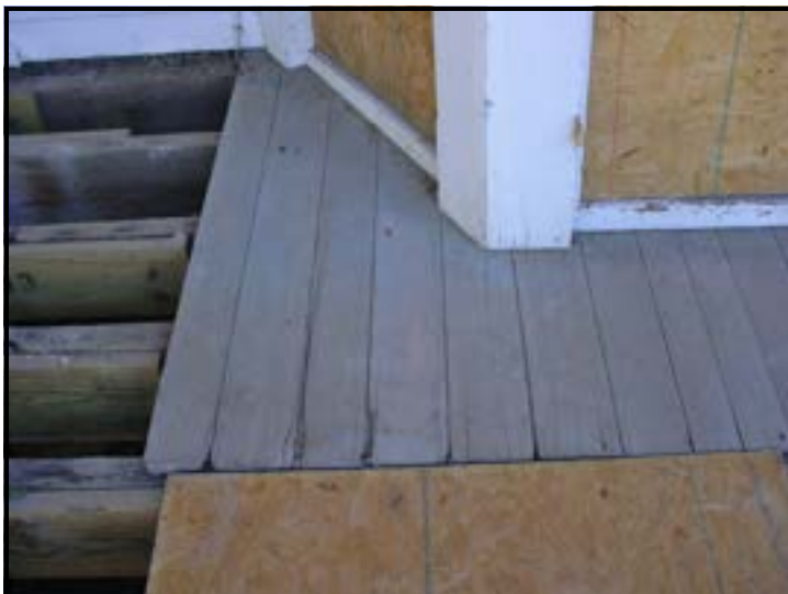
The photo at left shows the original tongue and groove flooring that was left around the bay window area of the ell porch.
