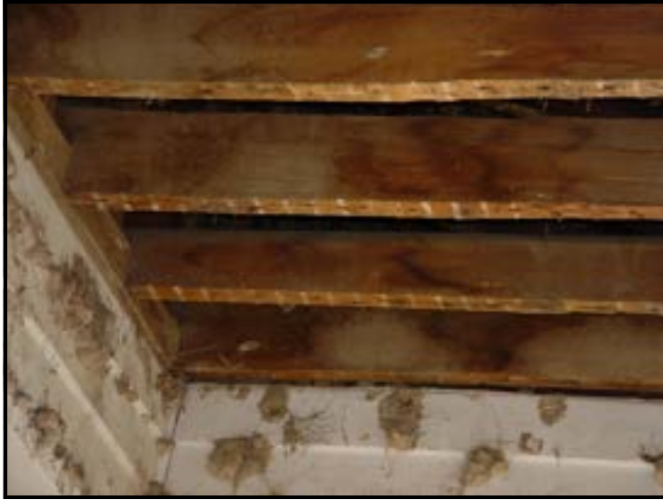
In the photo at left marks left by the original lathe and plaster ceiling can be seen. Evidence of the lathe and plaster ceiling was discovered when the second ceiling was removed from the ell porch.
