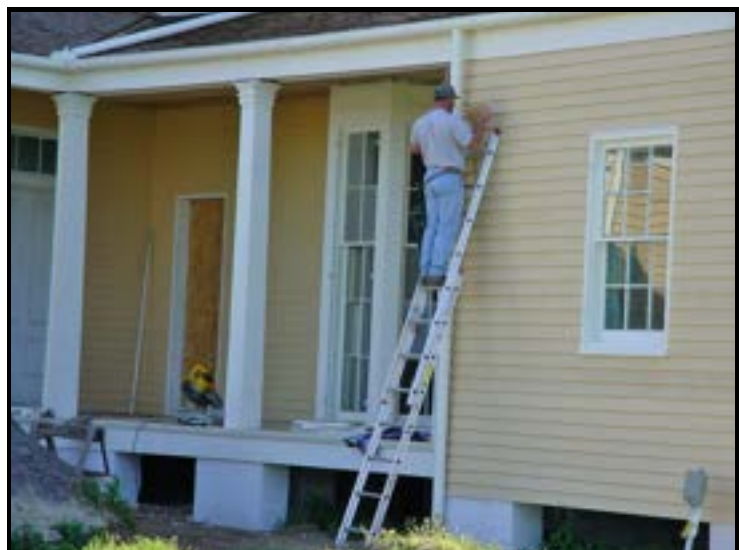
In the photo at right new columns have been constructed and set in place on the ell porch. The columns on the ell porch are built to match the columns on the front porch of Lakeport Plantation house
