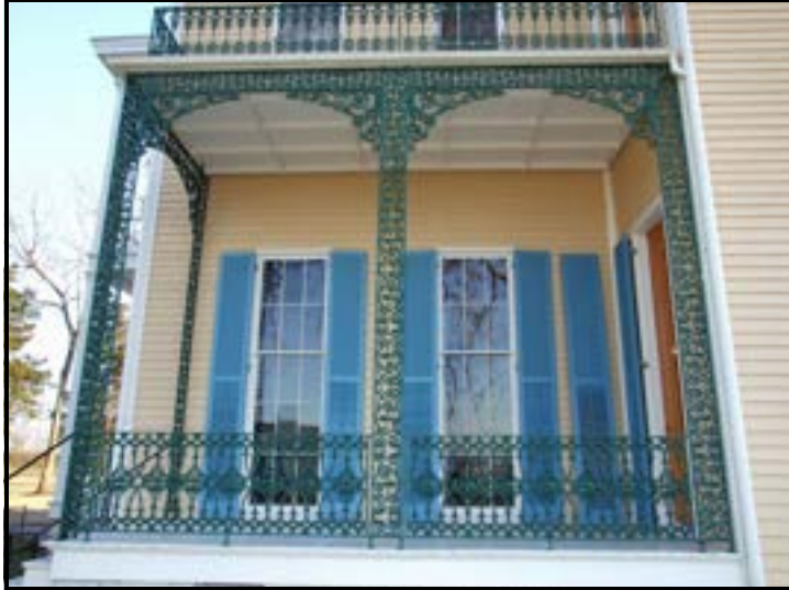
The ornamental iron porch is constructed almost entirely of decorative cast iron. It can be accessed from the north parlor. Because of its location and design, It is considered to be the more formal porch
