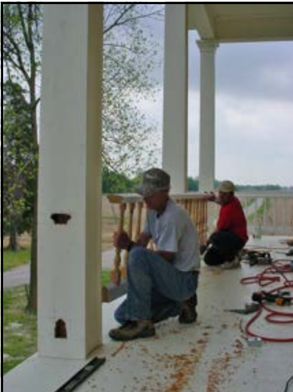
The photo at left shows restoration crew members setting a section of the new front porch balustrade into place.
