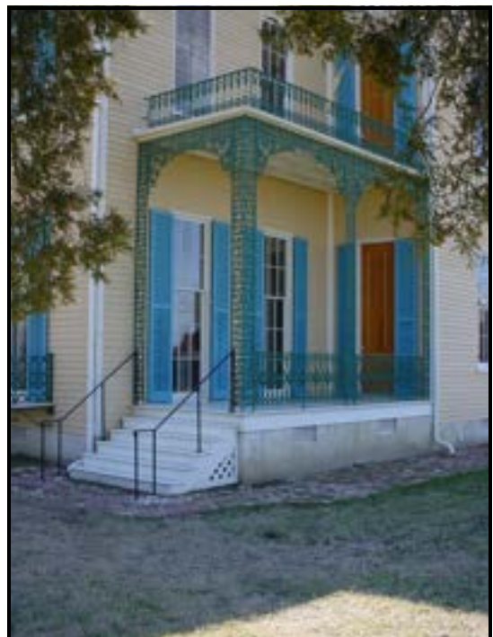
In the photo at right the ornamental iron porch has been completely restored to its original condition.
