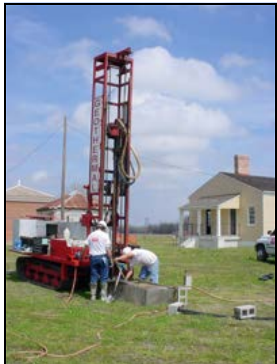
In the photo at right preparations are being made to begin digging the wells for the geothermal field for Lakeport Plantation house. A test loop had previously been dug and it was determined that, to maximize the thermal quality of the ground, each well would need to be three hundred and sixty feet deep with a distance of twenty-five feet between all wells.
