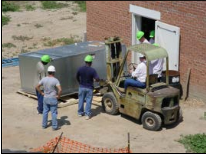
The photo at left shows the large air handler being maneuvered through the smokehouse door. Once inside, the air handler will be raised to the mezzanine floor where it will be installed.
