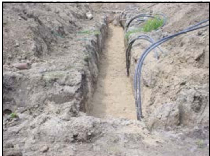
The photo at right shows a single row of five wells. What appears to be two pipes running into the ground for each well is actually one pipe that runs into the ground, loops below ground, and then comes up and out of the ground.
