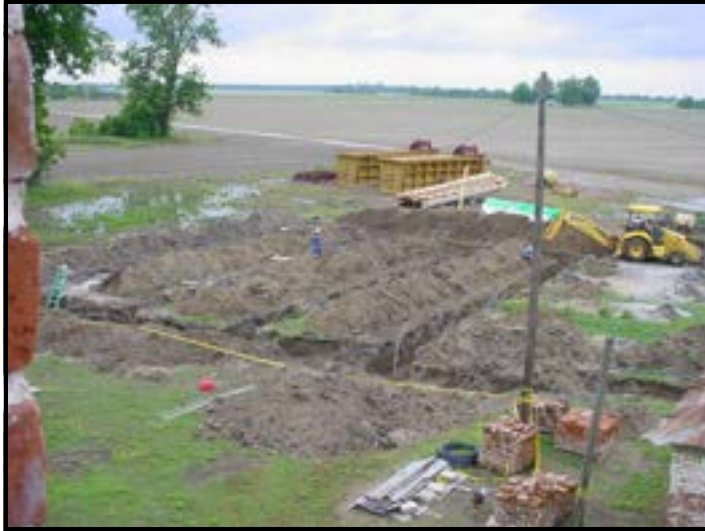
The photo at left shows an aerial view of the geothermal field as it is being dug for Lakeport Plantation house. The geothermal field consists of five rows of loops with five vertical loops, or wells, in each row.
