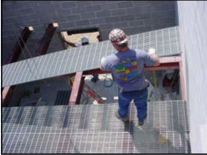
The photo at left shows the construction of the mezzanine floor in the new smokehouse. The mezzanine floor was necessary to be able to house all of the mechanical equipment in the smokehouse.
