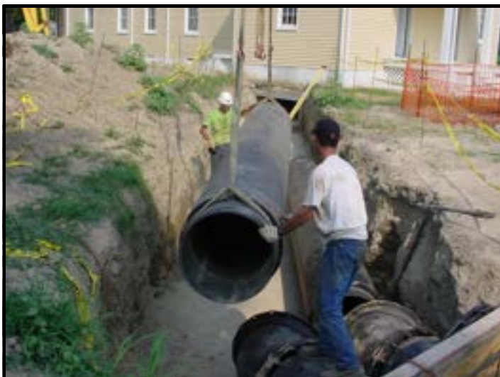
The photo at left shows the large cast-iron pipes being run from the smokehouse to Lakeport Plantation house. The large pipes are twenty-four inches in diameter.
