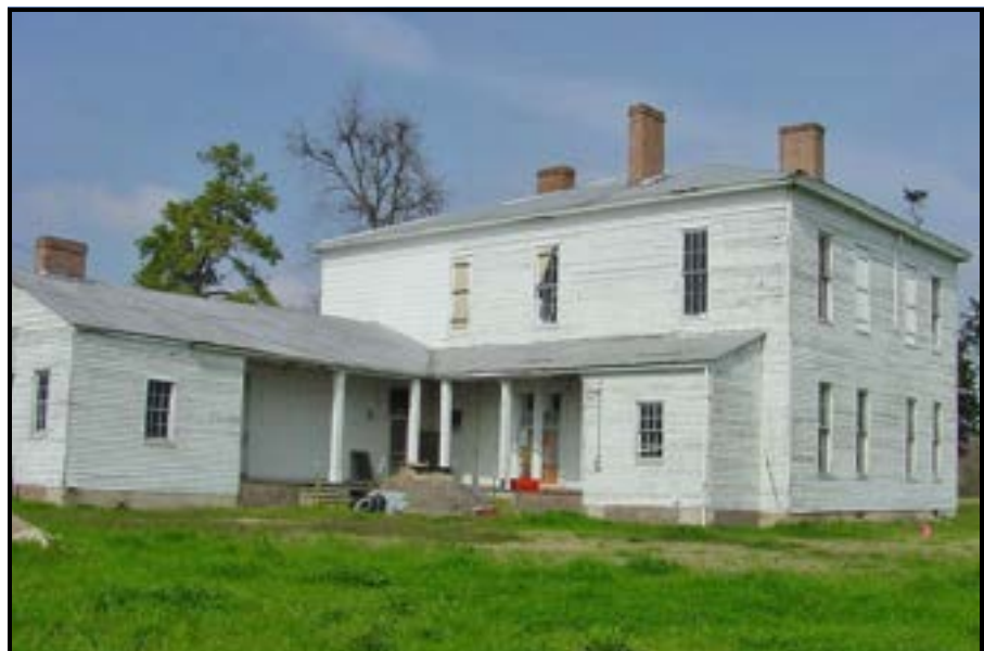
This photo of Lakeport Plantation house shows the four chimneys that were visible at the time restoration began. The fifth chimney had been taken down to below the roof line.
