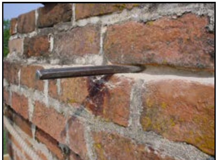
This photo shows the mortar being removed with a hand chisel. Power tools can damage historic brick and should not be used to remove mortar on historic masonry.
