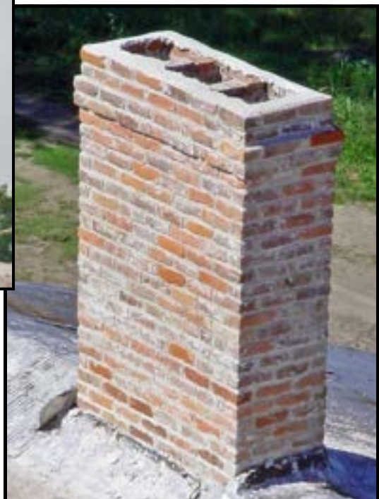
The photo above shows the west wing chimney being disassembled by a restoration crew member. Historic photos showed that the chimney had been shortened in previous years. Restoration plans were to disassemble the chimney and rebuild it to match the existing chimneys. The photo at right shows the chimney after being rebuilt.
