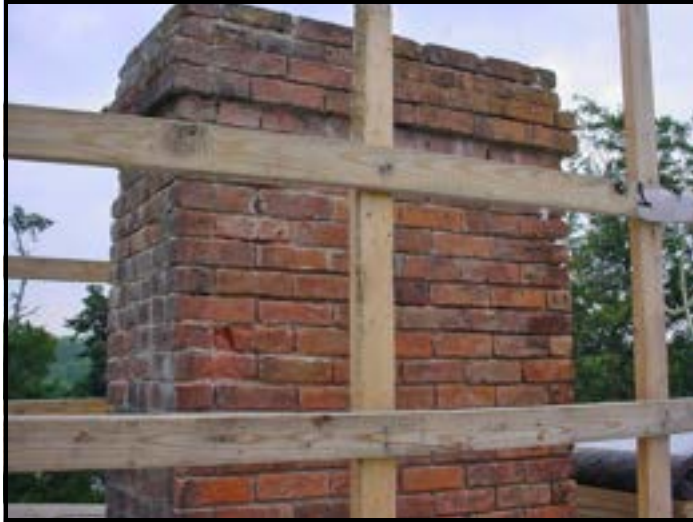
This photo shows the northeast chimney of Lakeport Plantation house after the mortar had been removed to prepare the chimney for repointing.
