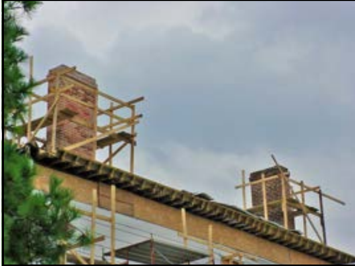
The photo at left shows a comparison of the southwest chimney on the right and the northwest chimney rebuild on the left. The northwest chimney had been taken down to below the roof line before restoration began. The photo below shows a closer view of the northwest chimney after being rebuilt.
