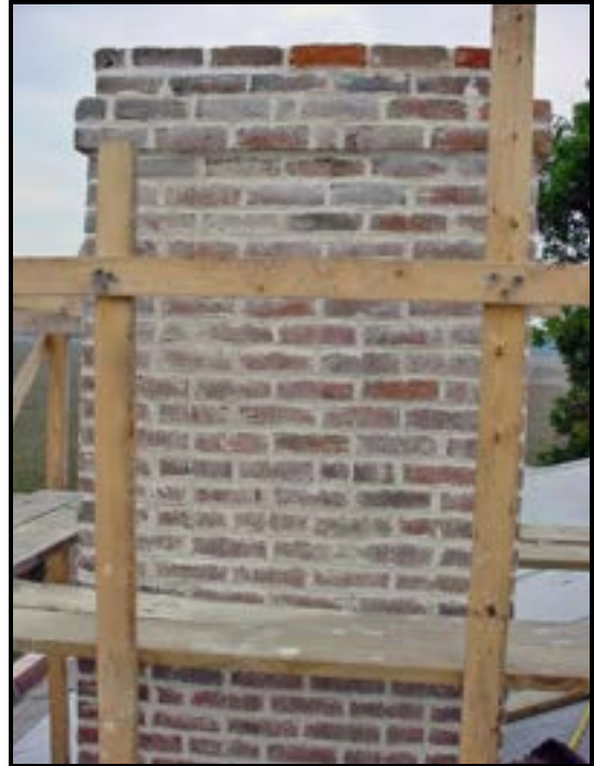
The above photo shows the southwest chimney after being repointed. A lime mortar compatible with the soft historic bricks was used to repoint the chimneys.
