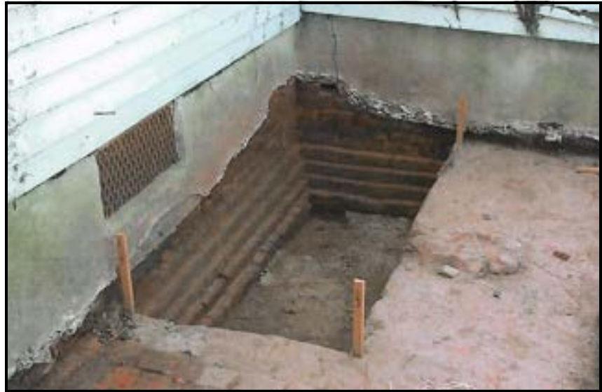
The photo above shows the corbelled brick footer that was uncovered by the archeologists during excavation of the grounds around Lakeport Plantation house. This photo was taken from the Historic Structures Report for Lakeport Plantation.
