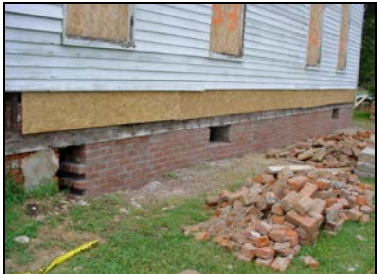
The photo at right shows a large section of the exterior foundation wall after being rebuilt. The brick piles are the original historic bricks that were disassembled and removed. The historic bricks were too deteriorated to be salvaged and reused.
