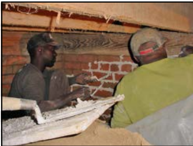
The photos at left and below show the brick masons working underneath the house, repointing mortar joints of the interior foundation walls. The mortar had deteriorated over the years and had to be removed and the foundation walls repointed.
