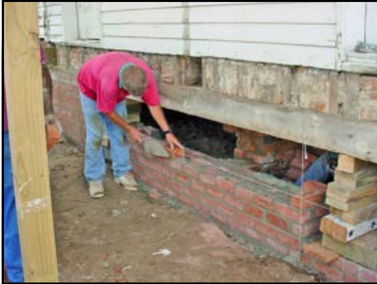
The photo at left shows a brick mason laying the new exterior foundation wall. The foundation walls are three bricks thick and ten courses high and set on top of the footers. There are foundation walls to support all interior as well as exterior walls.
