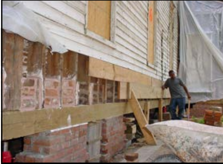
The photo at left shows a large sill beam that has been replaced, resting on top of the partially rebuilt foundation wall of Lakeport Plantation house. The sill beams support the floor joists and walls of the house.
