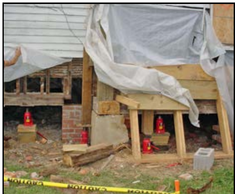
The photo at right shows the framing of Lakeport Plantation house being supported with hydraulic jacks and kicker boards during removal of the exterior foundation walls. The foundation walls were disassembled in short sections and rebuilt using reproduction "handmade" bricks.
