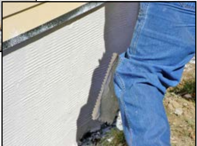
The photo at right is a close-up of the scratch coat after being raked or "scratched".
