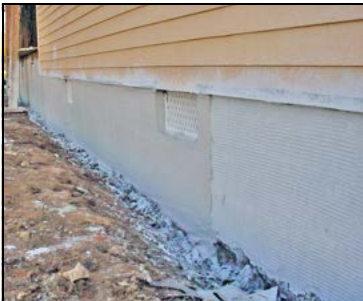
The photo at left shows a view of the scratch coat and brown coat applications side by side. The photo above shows an up-close view.
