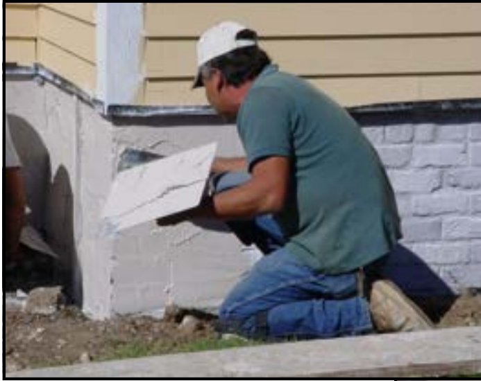
The photos at left and below show the scratch coat being applied to the foundation walls of Lakeport Plantation house.
