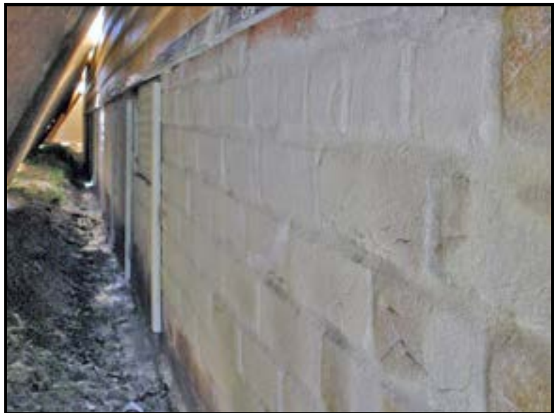
This photo shows the foundation walls of Lakeport Plantation house after the limewash was applied. Notice how the walls have been covered with sheets of plywood to protect the limewash from the sun to prevent quick drying.
