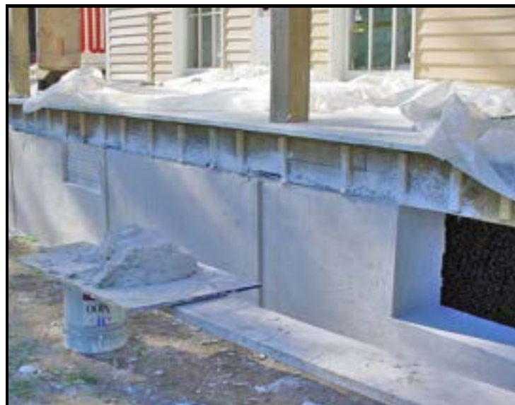
The photo at left shows a view of the scratch coat and brown coat applications side by side. The photo above shows an up-close view.
