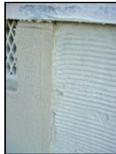
The photo at left shows a view of the scratch coat and brown coat applications side by side. The photo above shows an up-close view.
