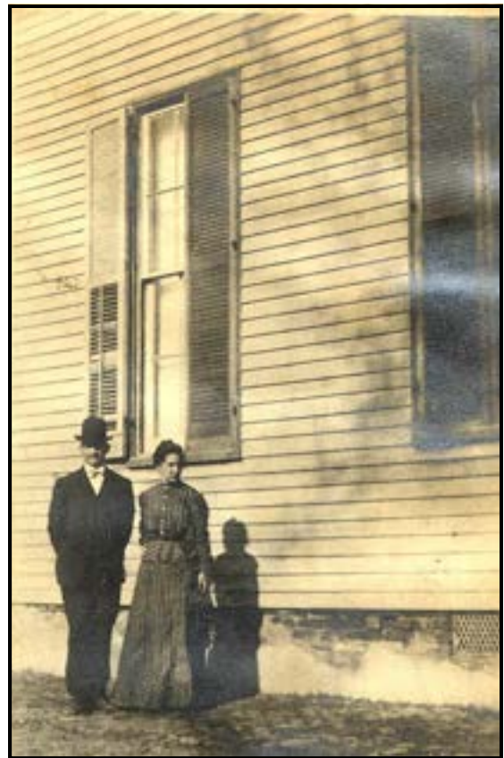
This photo of Lakeport Plantation house, taken during the early 1900's, shows the original parge coating on the foundation walls. This photo was provided by descendants of the Johnson family.
