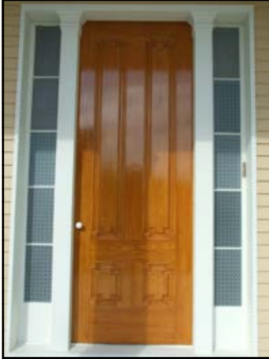
This photo shows the front entry door of Lakeport Plantation house with the decorative glass sidelights. Three of the original glass panes remain. Reproduction glass panes were made and installed where the original were missing.
