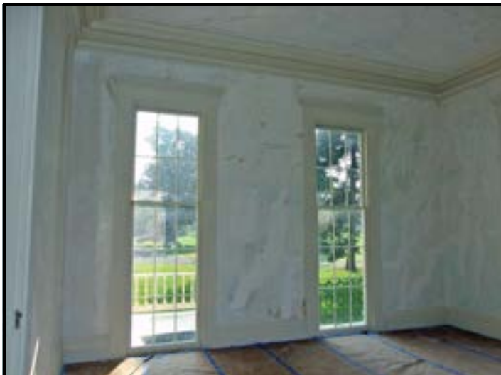
The interior window casings and head jamb, shown here in the north parlor, are simple but elegant.
