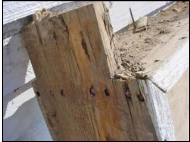
The photo at left shows the original window framing as it was being removed from the west wall of the kitchen. Below is a close-up of the window construction. Notice the mitered corners of the window framing. This type of construction is used to protect the end grain of the wood from absorbing moisture.
