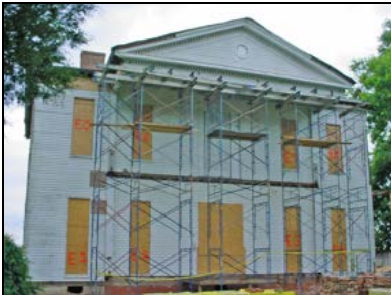
This is a photo of Lakeport Plantation house after all of the window sash were removed and taken to a window restoration expert for restoration.
