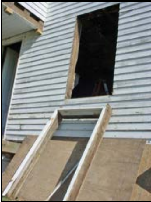
The photo at left shows the original window framing as it was being removed from the west wall of the kitchen. Below is a close-up of the window construction. Notice the mitered corners of the window framing. This type of construction is used to protect the end grain of the wood from absorbing moisture.
