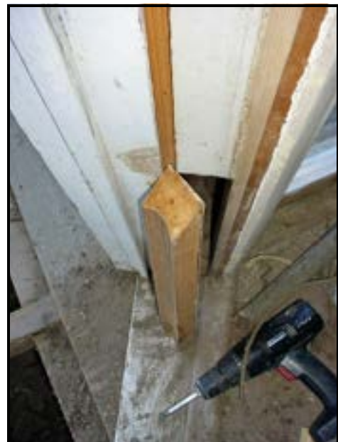
The photo at left shows the window pocket which houses the window weight for the bay window at the back of Lakeport Plantation house. The pocket runs the length of the window to allow the weight to move up and down as the window is raised and lowered. The photo at right shows the pocket door which provides for easy access to the window weight when repairs are necessary.
