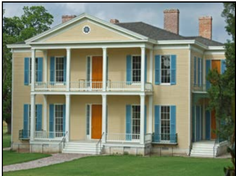
The tall, symmetrical windows of Lakeport Plantation house help to define the Greek Revival architectural style of the house.
