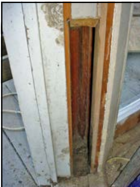
The photo at left shows the window pocket which houses the window weight for the bay window at the back of Lakeport Plantation house. The pocket runs the length of the window to allow the weight to move up and down as the window is raised and lowered. The photo at right shows the pocket door which provides for easy access to the window weight when repairs are necessary.
