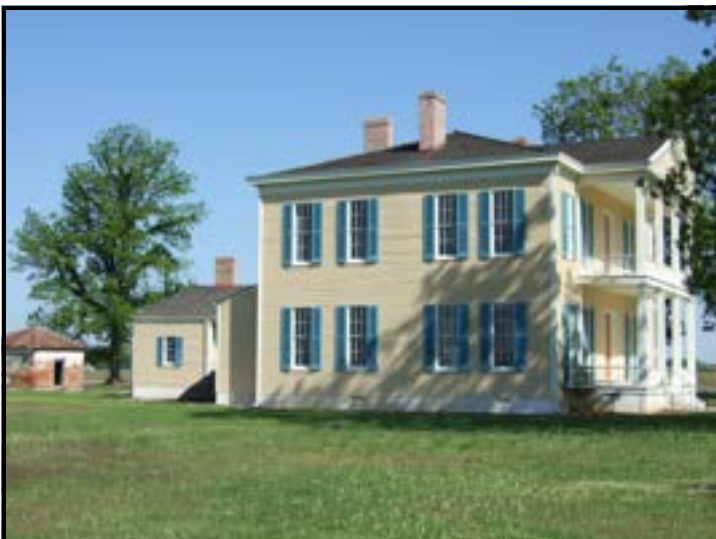
This photo shows the south side of Lakeport Plantation house after window restoration is complete and the shutters have been hung. Often referred to as the "eyes" of the house, windows are one of the most important architectural features of a house.
