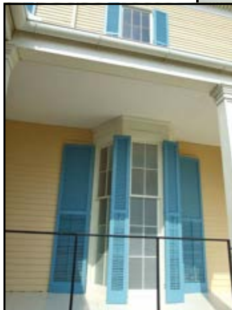
Before and after photos of the bay window at Lakeport. Many panes of decorative glass are original. Reproduction glass replaces any missing or broken panes.
