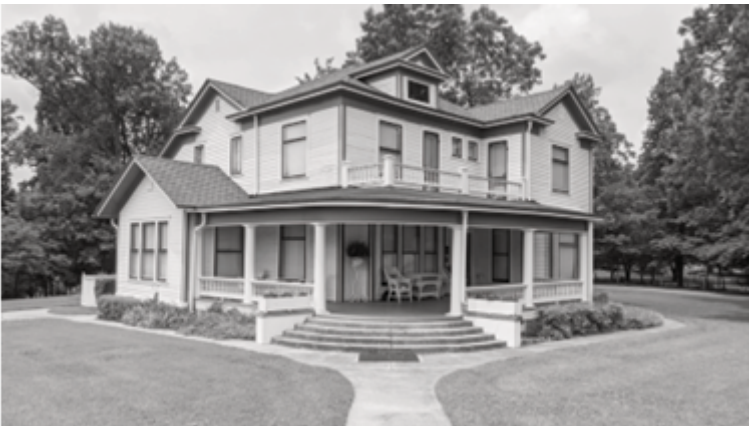
Hemingway-Pfeiffer House. Photo courtesy of Damon Guinn.
